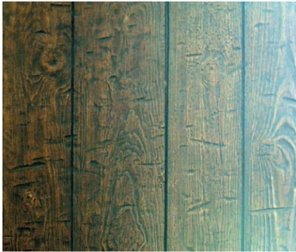
Figure 28-2 Antiqued Paneling The New Old The indentations that suggest age can be felt as well as seen in this antiqued plywood paneling used as an accent wall.
