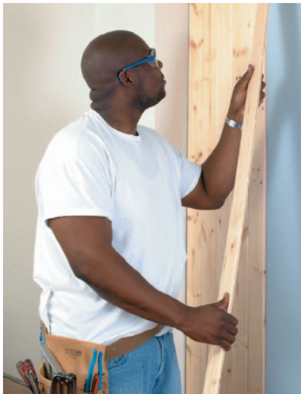
Figure 28-9 Installing Board Paneling
